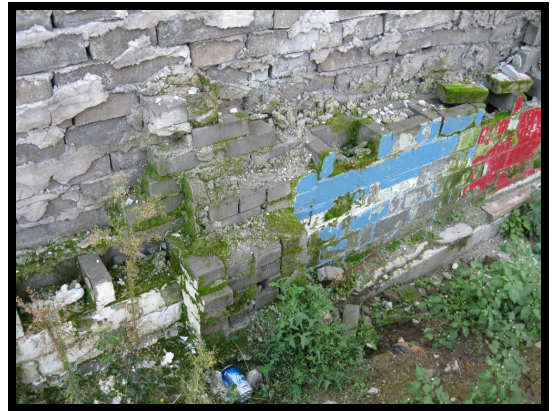
Close up of lead paint on bricks
