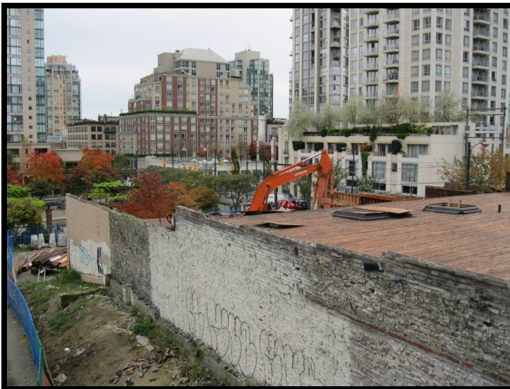
Building tear down
