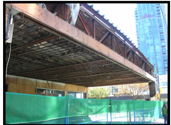
Engineered demolition of canopy at property lines
