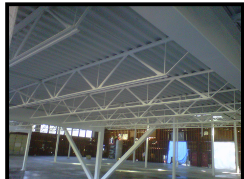
Completed project - Following paint encapsulation
