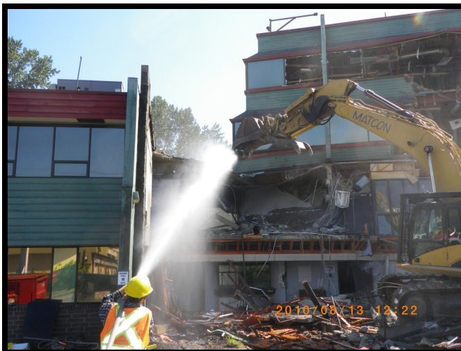
Building separation & four-storey tear down
