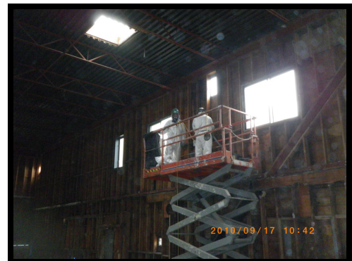
Wood members vacuumed with HEPA vac
