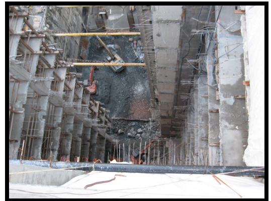
View of removed floor structure from above
