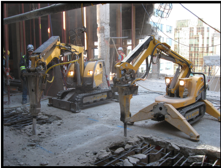
Structural demolition using robotic equipment
