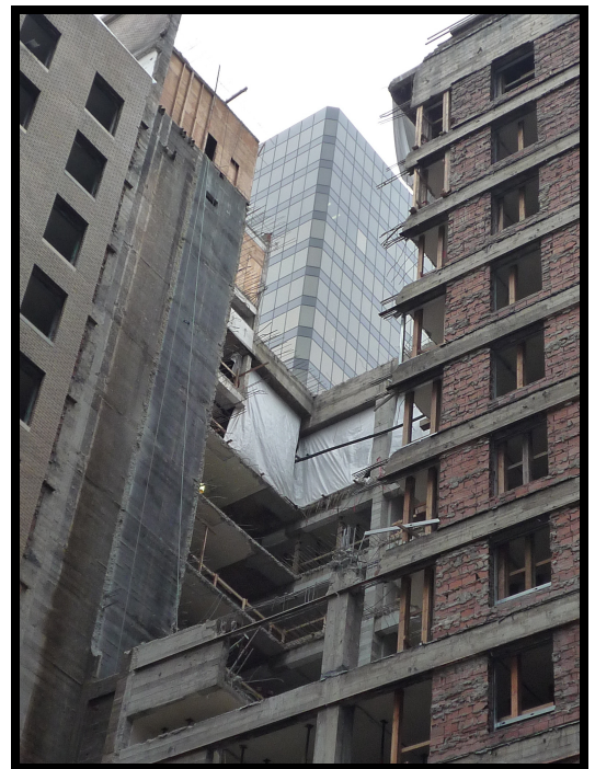
View of removal structure from below
